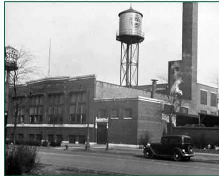
*Calumet Refining Company formed in Burnham, IL (1919)
